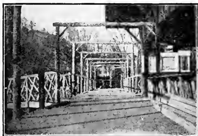
NEW BRIDGE LEADING FROM STATION TO ASSEMBLY GROUNDS.
